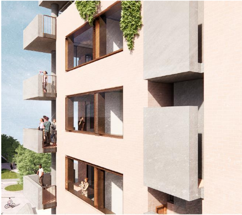
Figure 79: Drying court walls are integrated into building architecture and to be constructed using pre-cast concrete
