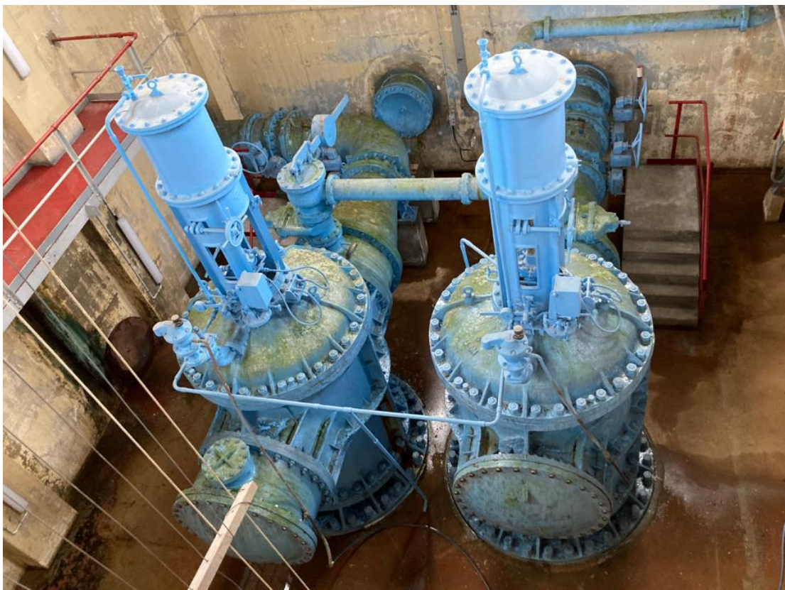
Figure 12: Internal view: Valve House
