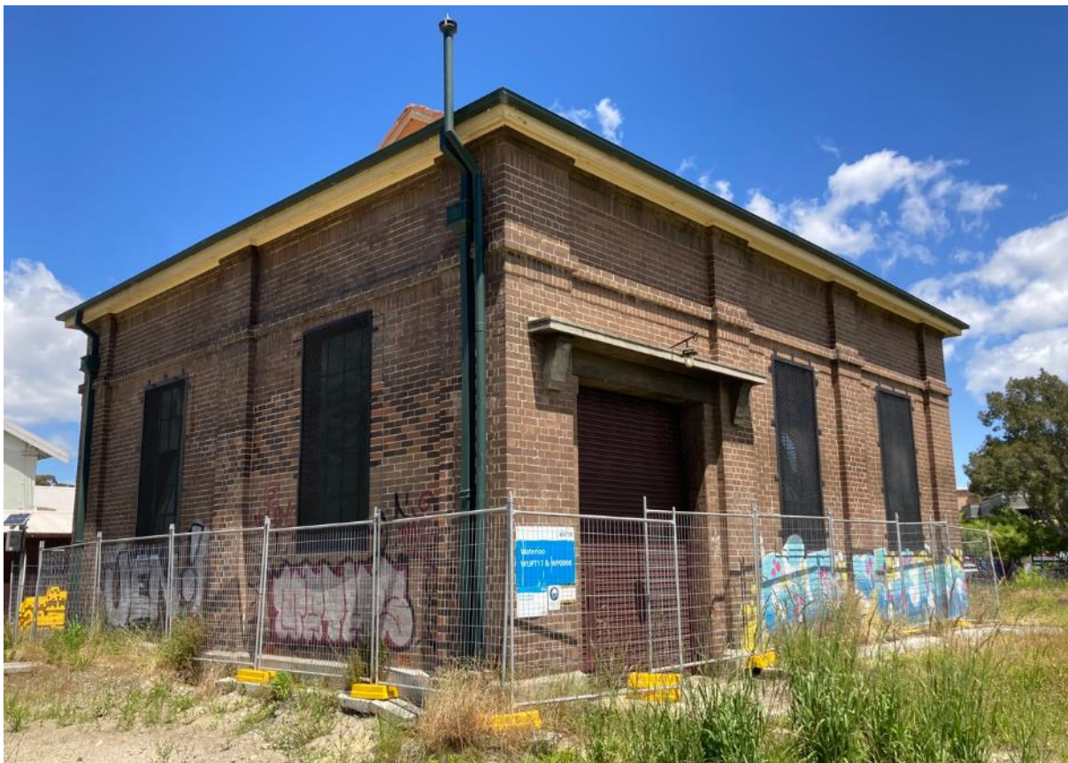
Figure 8: Valve House (northern facade)
