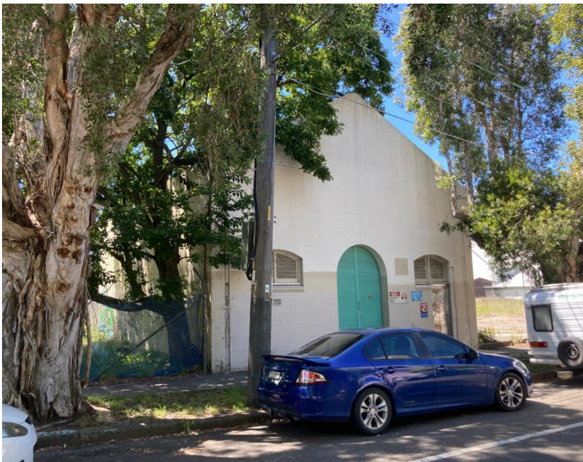
Figure 6: Substation within the curtilage of the site, viewed from Young Street, generally looking east
