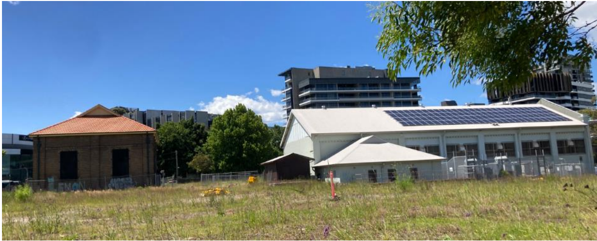
Figure 7: Site buildings, including the Valve House (left) and Pump House (right), viewed from Young Street, looking east
