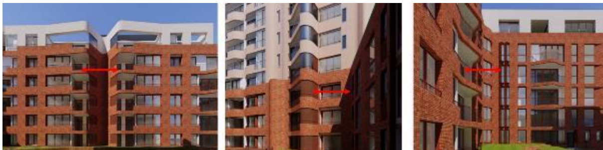
Figure 83: Angled privacy screens have been provided to prevent direct mutual overlooking and windows are angled to prevent overlooking of neighbouring apartments (red arrows)
