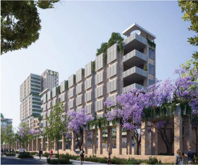
Figure 66: Photomontage, extracted from the Competitive Design Alternatives Report for D1(a) and D1(b), showing an arbor to Young Street and external, shade devices that have been redesigned for the western elevation of the Young Street Buildings
