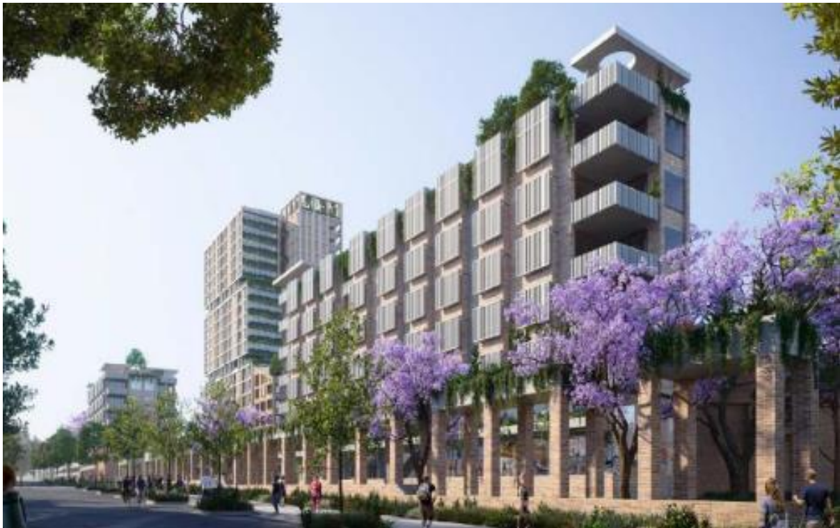
Figure 16: Photomontage from the Competitive Design Alternatives Report for D1(a) and D1(b). The masonry arbor shown in the image above has been removed and external masonry shade devices have been redesigned for the western elevation of the Young Street Buildings.
