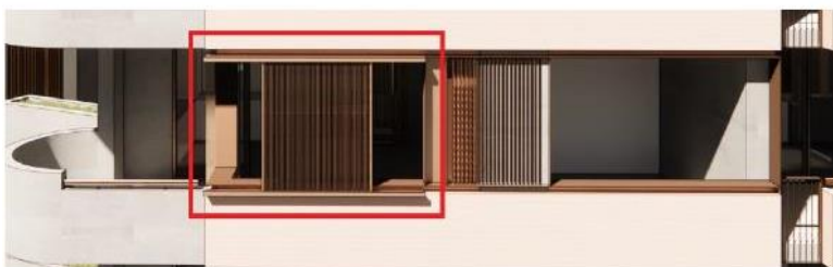
Figure 69: External, operable sunscreens for Young Street Buildings that are less visually dominating than those shown for the winning design scheme (Figure 66 above)
