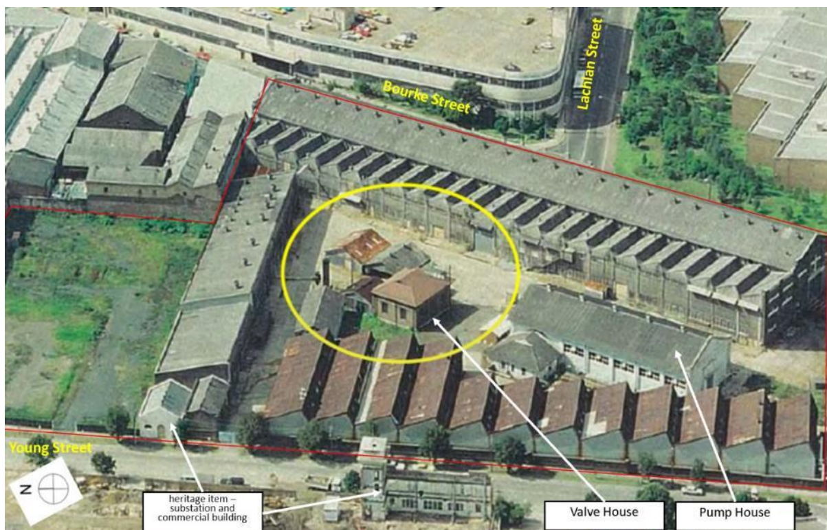
Figure 13: Historic aerial photo (c.1989) of site showing maintenance buildings on site (now demolished), heritage listed buildings, including the Pump House, Valve House (circled in yellow), substation and commercial building at Young Street. Source: heritage impact statement.
